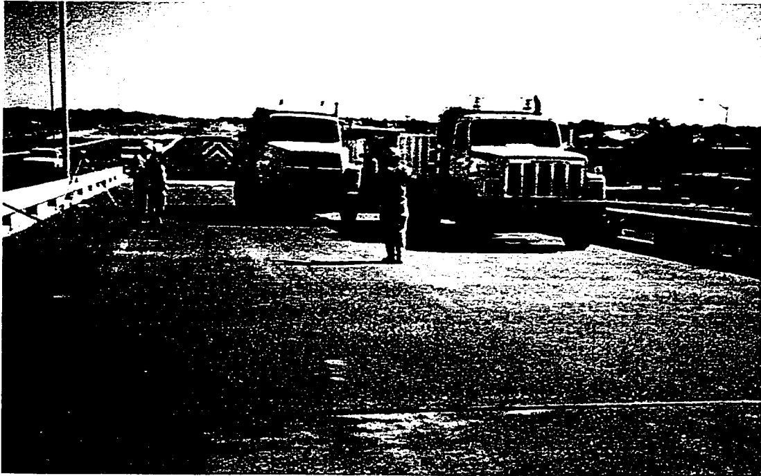
Figure 9.1 - Test Trucks Being Positioned During San Angelo Live Load Tests
