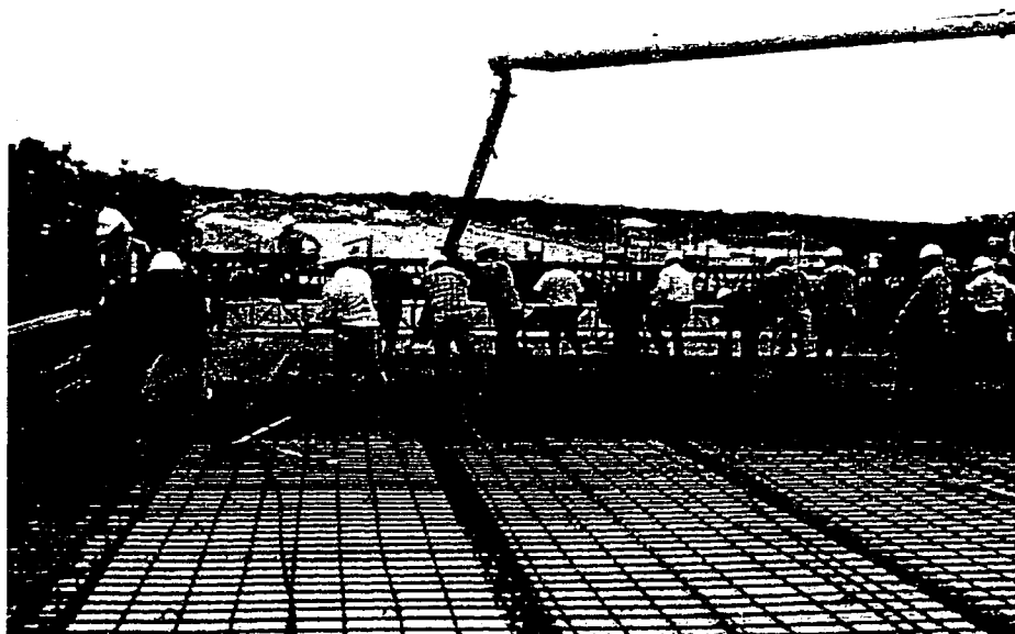
Figure 2.29 - Deck Placement in the Eastbound Bridge
